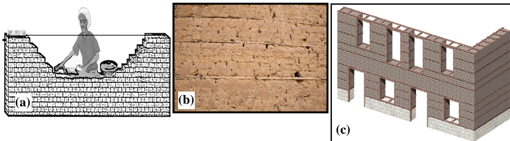
Fig. (5): Timber-tie system in masonry construction: a) A sketch of building contemporary brick-walls , b) 3D-view of adobe dwelling with timber ties, Greece, c) Adobe wall and timber ties, Greece, (b & c after: Vissilia, A. and Villi, M., 2010: p.301).
