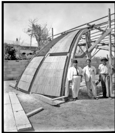
a) Trying the cutting out of lead plates for covering dome surfaces.
