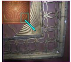
Fig. 13 Photographs (macro and micro) corresponding to the ceiling extension of mosque of palace of prince Mohamed Ali (previous gilding intervention) shows the severe damage.
